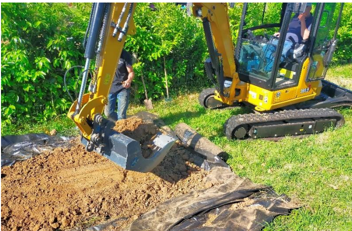
In depot leggen van bodem met worteldelen
