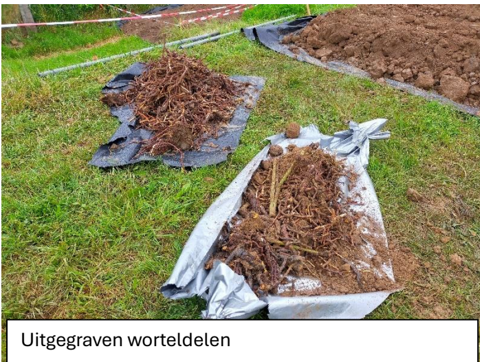
In depot leggen van bodem met worteldelen
